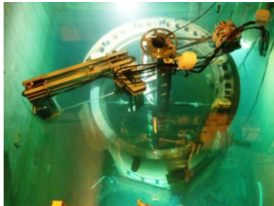
Figure B.12. Remotely operated bandsaw for internals segmentation at Jose Cabrera
