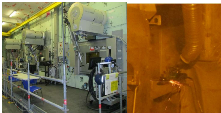
Figure B.43. Top, ELAN 2B dismantling workshop achieved using a combination of 3 telerobots paired with 3 mechanical telemanipulator MT200. Bottom, the results obtained in cutting tasks.
