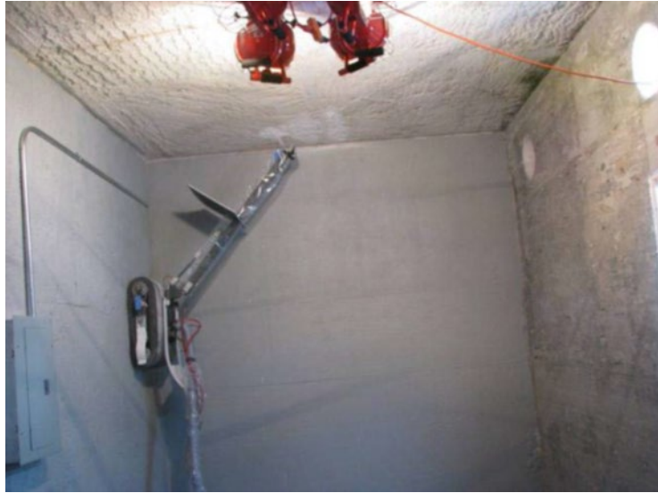
Figure B.4. ICM climbing machine spraying fixative
