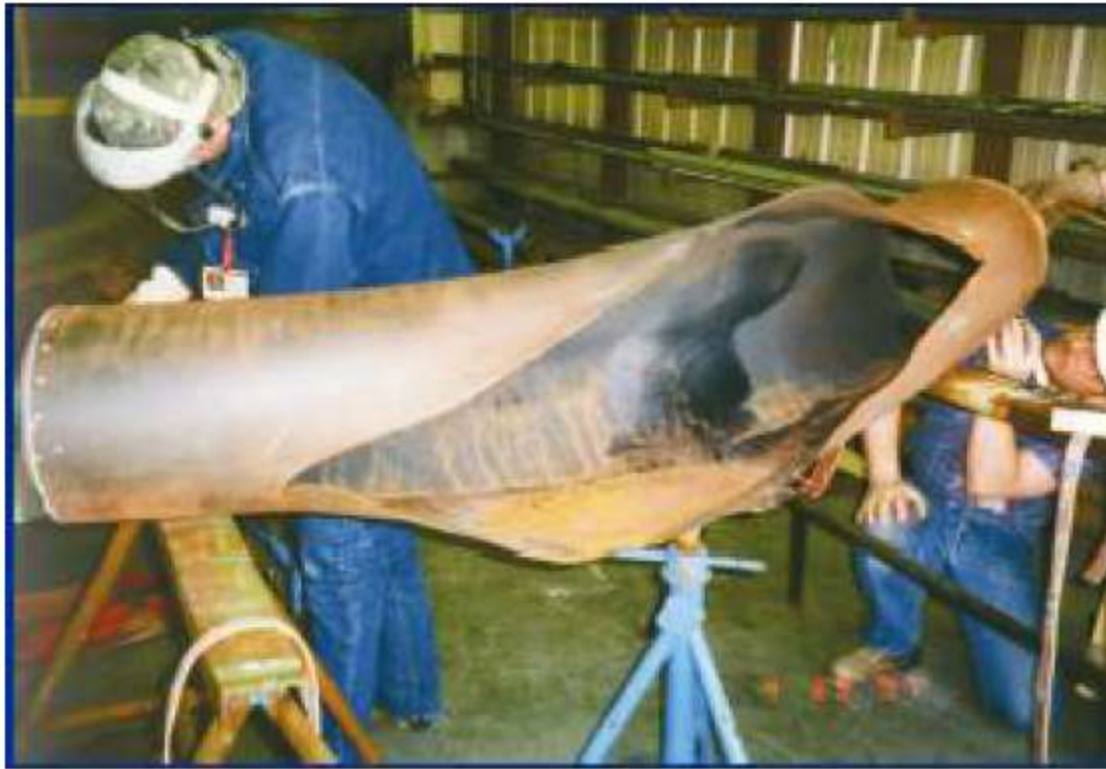
Figure A-2: Ruptured Long-Radius Elbow
