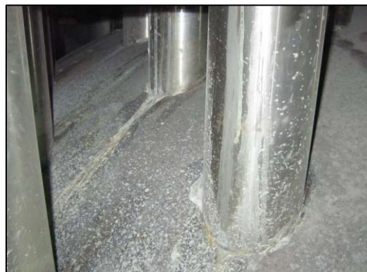
Reactor Vessel Head
