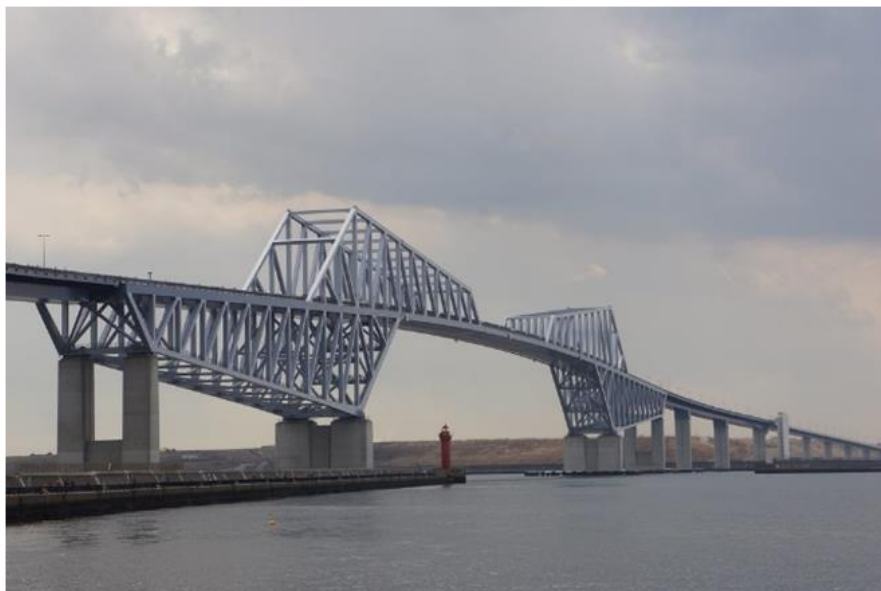
Figure 2.1. Fluoropolymer Paint Application in Bridges
